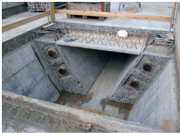
Fig. 5 Typische Abspannstelle. Typical anchoring of prestressing tendons.
