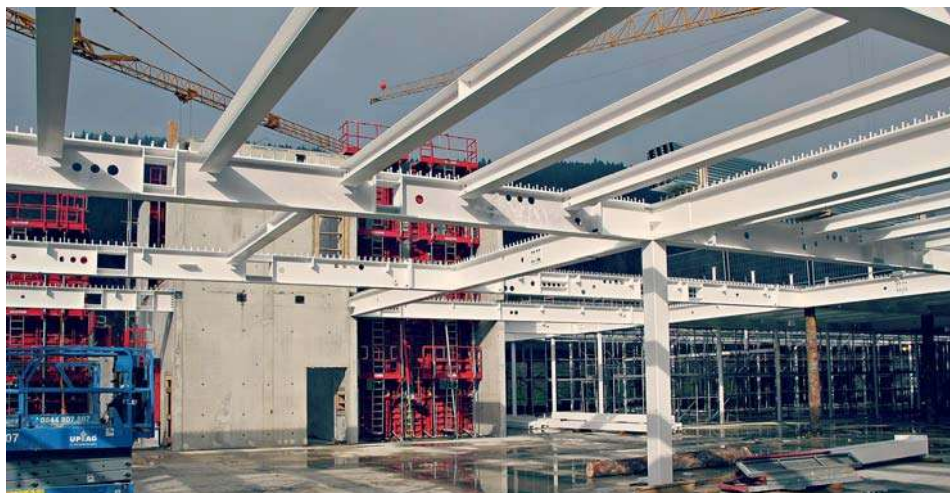
Fig. 3 Montage de la charpente sur atelier. Assembly of the roof structure on the workshop.
