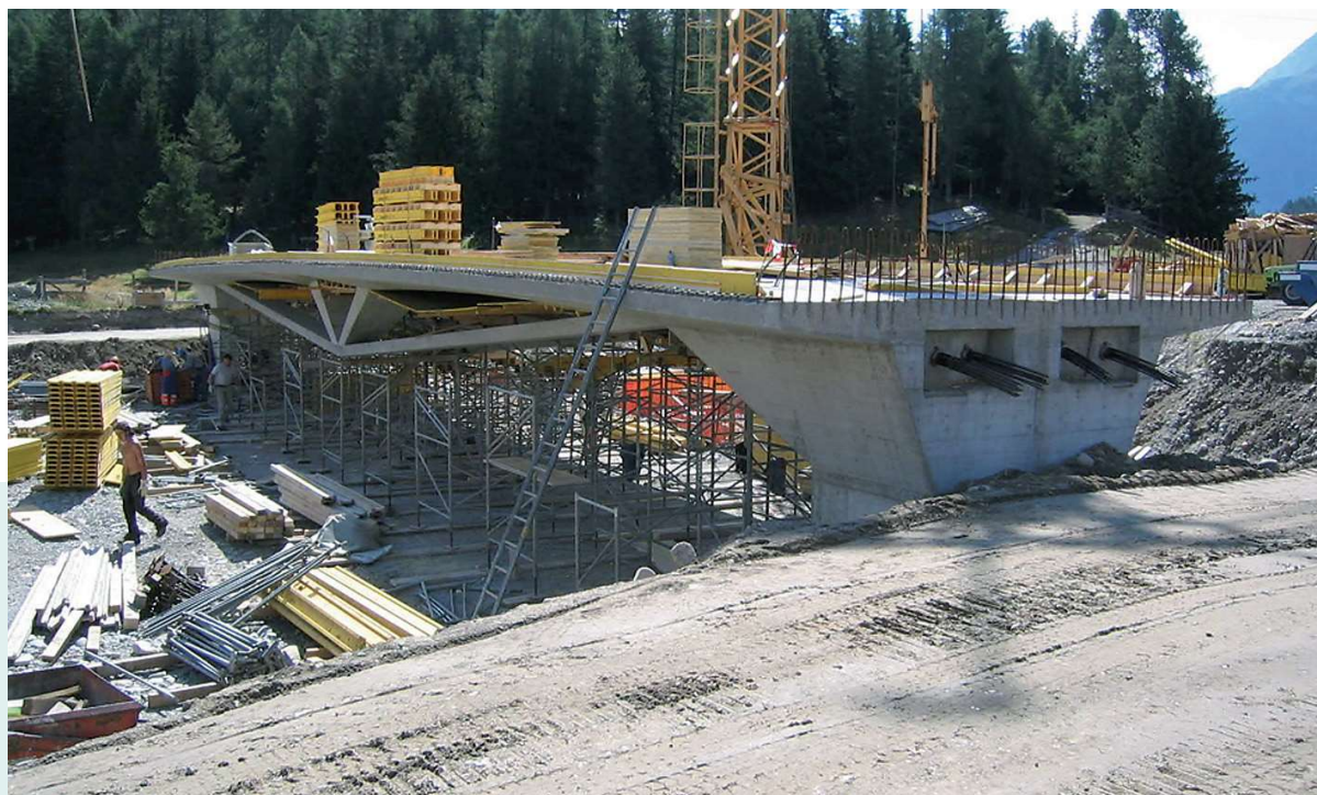
Vista del Ponte Pradé in costruzione General view of Pradé Bridge in construction
